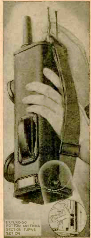
Antenna switch detail.
