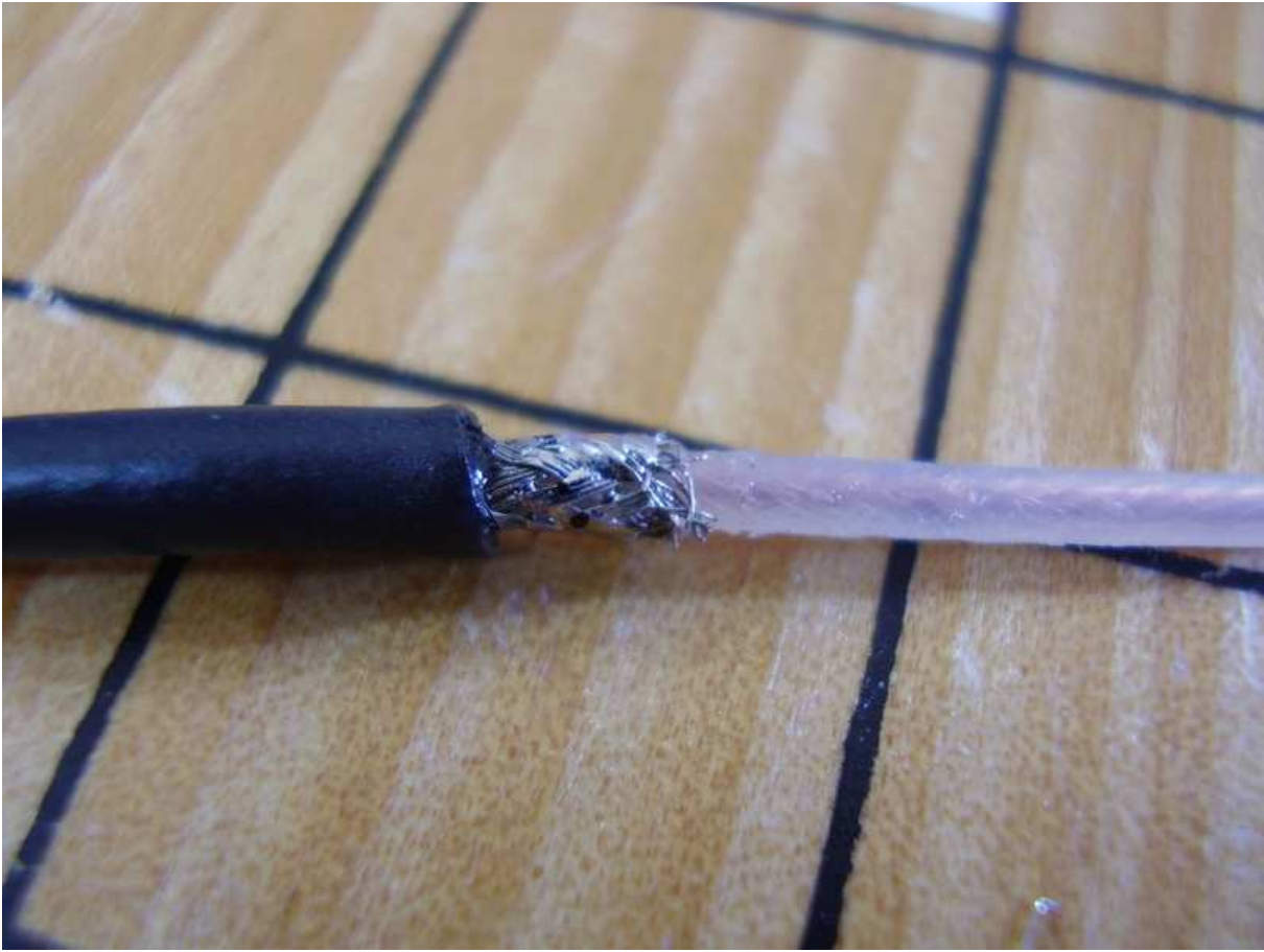
Figure 11.3: Remaining Shield Removed.
